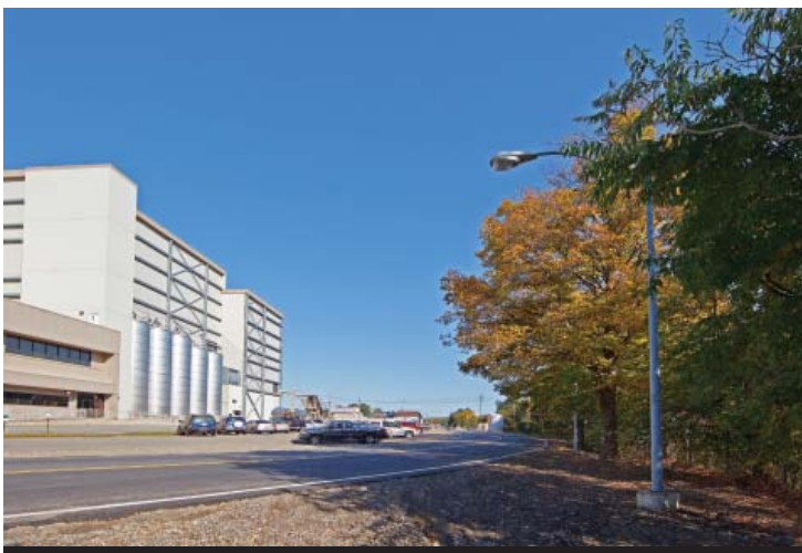
Yanuzzi Drive has been reconfigured for safer and more efficient access to and from the Leprino Foods plant in South Waverly.
