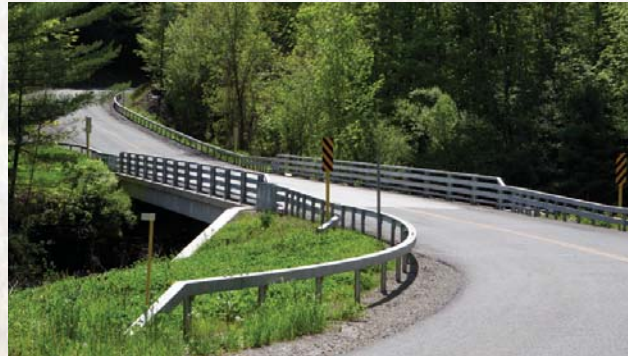
The Van Zandt Hollow Bridge across Glen Creek.
